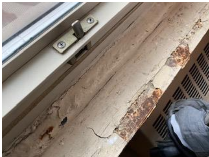
Interior Apartments. Metal Window Sills and Casings (Original to Building) with mostly Intact LBP (Some metal casings are deteriorated and need stabilized). Drywall and Plaster around windows tested negative for LBP.
