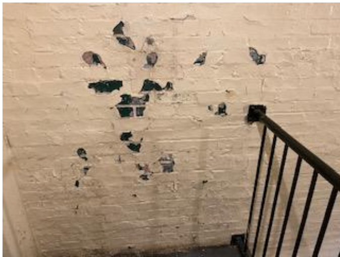
Interior Common Areas (Only Stairways). Brick Walls and Concrete Support Columns and Beams with LBP. Deteriorated Walls only found in 1314 Building, NE Stairway, 6 th Floor.
