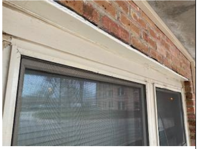
Exterior Building. Metal Lintels (over Doors and Windows) with Intact LBP.
