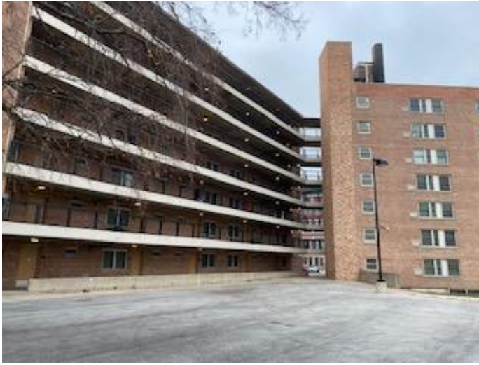
Exterior Building. Metal Hallway Fences with Intact Lead Based Paint (LBP).
