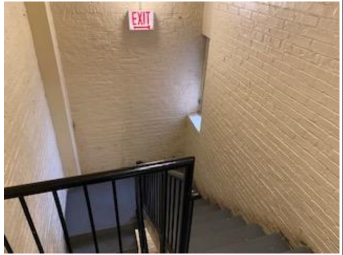
Interior Common Areas (Only Stairways). Brick Walls and Concrete Support Columns and Beams with Intact LBP.
