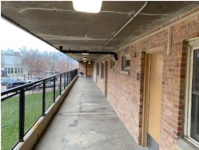
Exterior Building. Metal Hallway Fences and Lintels (over Doors and Windows) with Intact LBP.
