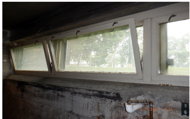
4. Typical basement vinyl hopper windows
