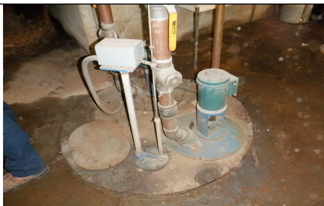
13. Basement sump pump
