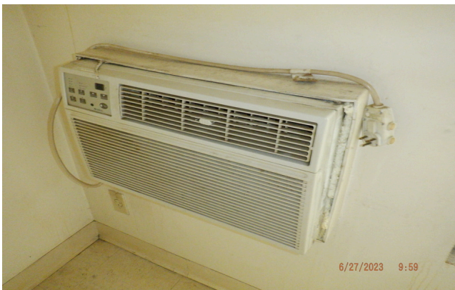
5. Typical unit through-wall air conditioning unit
