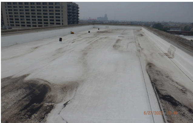
3. Typical TPO roofing
