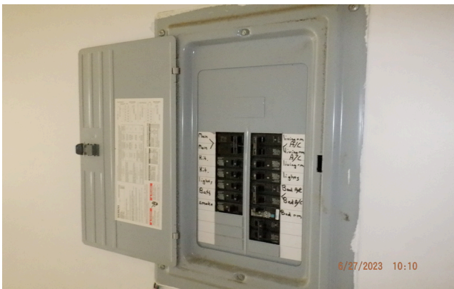
11. Typical unit electrical panel
