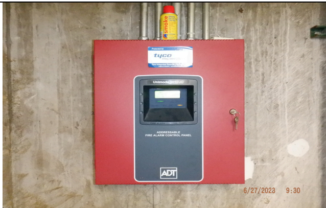
1. Fire alarm control panel
