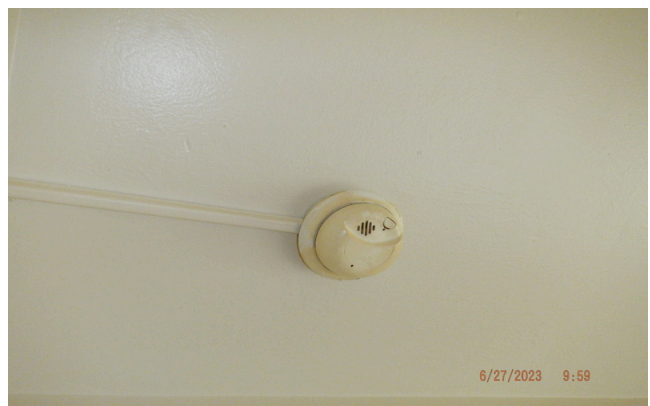
6. Typical hard-wired smoke detector
