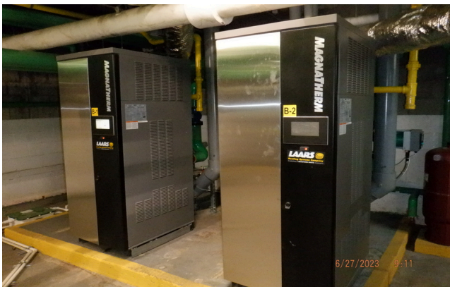
3. Radiant heat boilers
