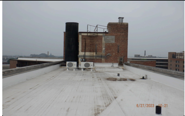
2. Typical TPO roofing
