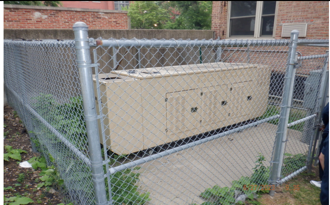
8. Gas-fired emergency generator
