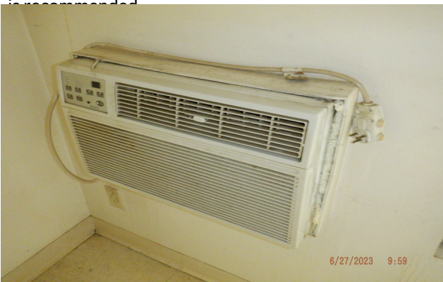
5. Replacement of through-wall air conditioning units is recommended at the end of their useful lives.
