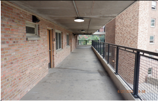
7. Typical elevated exterior concrete walkway with metal railings
