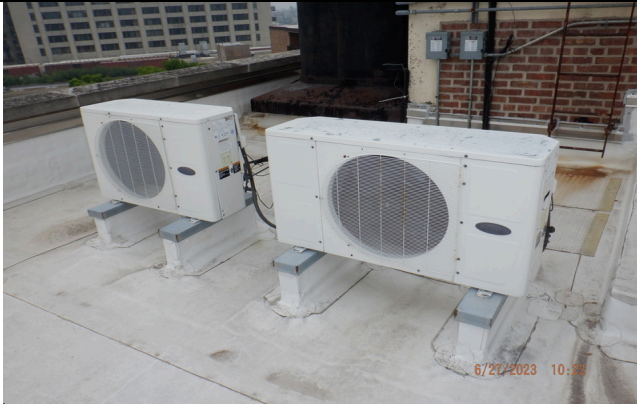
7. Elevator mechanical room mini-split condensing units
