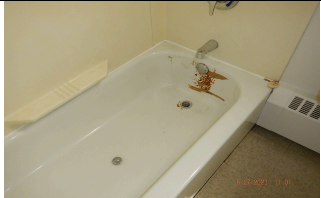
14. Hole in bathtub was observed in Building 1342 Unit 505. Repair is recommended.
