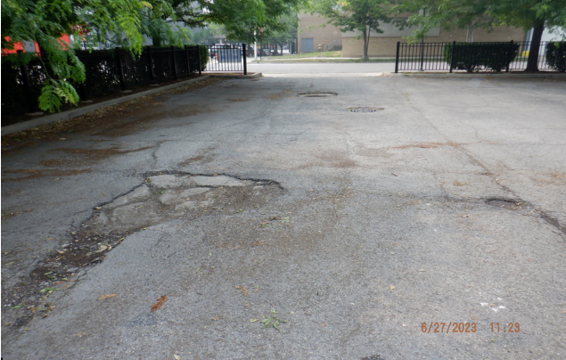
1. Mill, overlay, and restripe asphalt parking lots. Asphalt sealcoating is recommended every 5 years.
