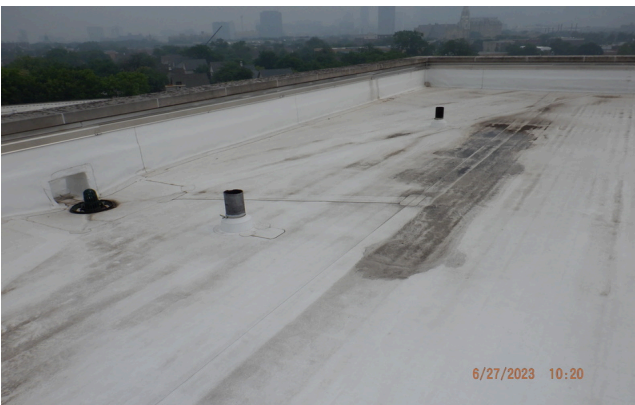
3. Identify and repair roofing leaks. The TPO roofing is approaching the end of its useful life and replacement is recommended.
