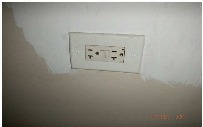
12. Typical GFCI receptacle
