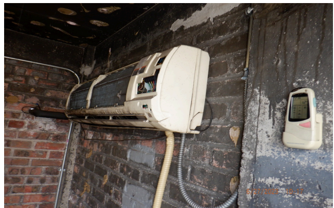
6. Elevator mechanical room mini-split air handler
