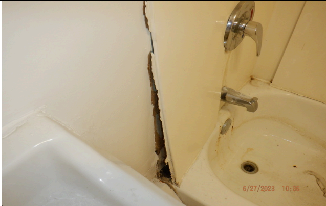
7. Water damage resulting from plumbing leaks was observed in both buildings. It is recommended that a plumbing contractor be engaged to perform
