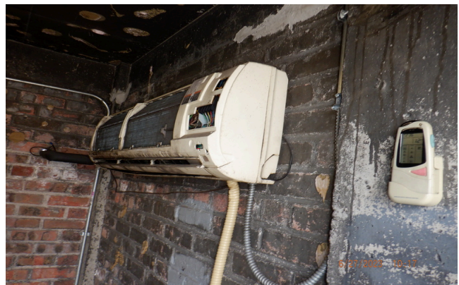
6. The mini-split ductless air conditioning systems servicing the elevator mechanical rooms are not operational. These units should be repaired or replaced.
