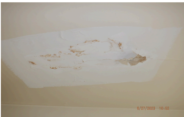
11. Roof leak observed in Building 1342 Unit 705. Repair is recommended.
