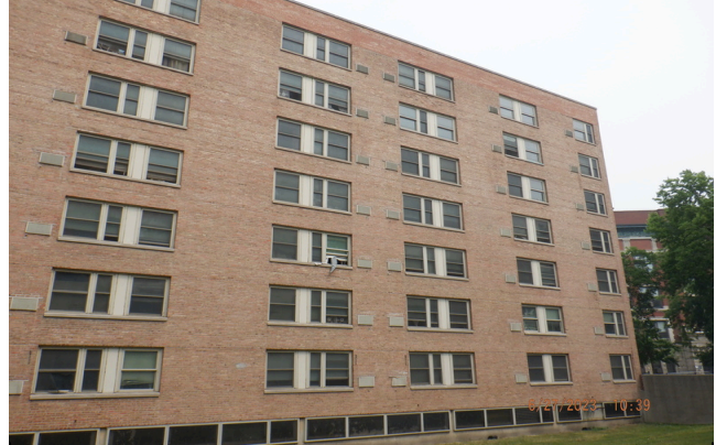
2. Selective repairs to the brick facade and tuckpointing are recommended.
