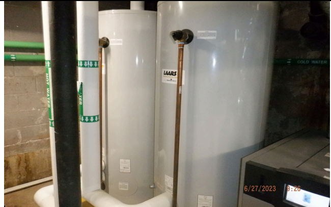
2. Hot water storage tanks
