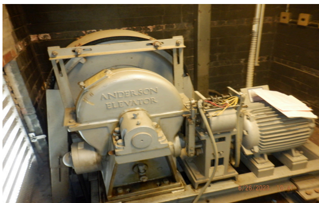
5. Electric traction elevator hoist equipment
