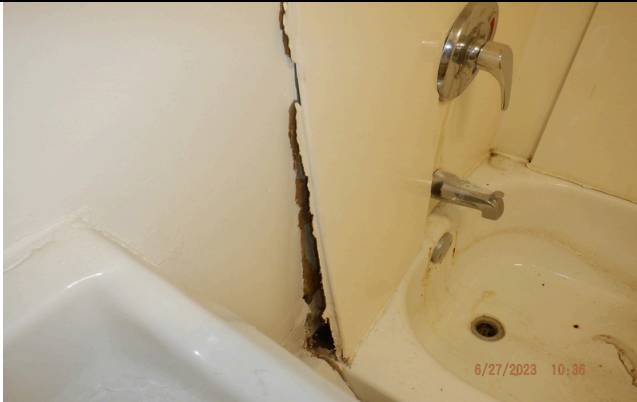
13. Plumbing leak in bathroom was observed in Building 1314 Unit 104. Repair is recommended.
