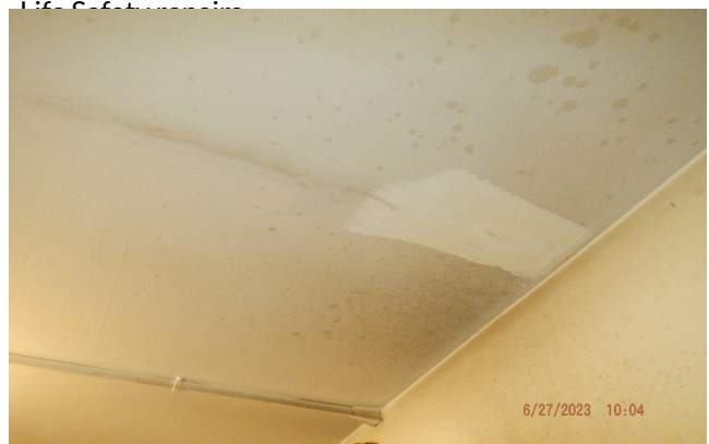
10. Roof leak observed in Building 1314 Unit 604. Repair of leak is recommended.
