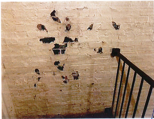
Interior Common Areas (Only Stairways). Brick Walls and Concrete Support Columns and Beams with LBP. Deteriorated Walls only found in 1314 Building, NE Stairway, 6 th Floor.
