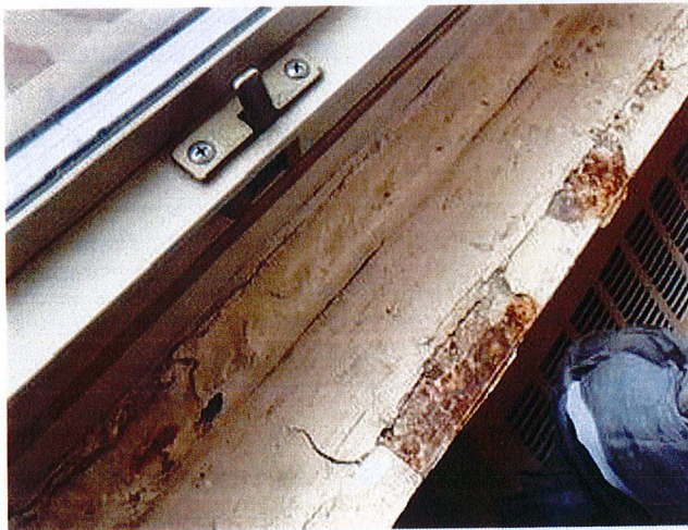
Interior Apartments. Metal Window Sills and Casings (Original to Building) with mostly Intact LBP (Some metal casings are deteriorated and need stabilized). Drywall and Plaster around windows tested negative for LBP.
